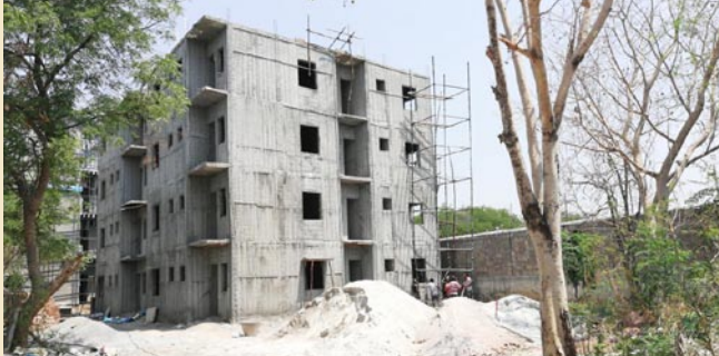
Gachibowli, Hyderabad, Telangana [32 DUs (G + 3)] using Structural Stay in Place Formwork System (coffor) - 16 DUs and Light Gauge Steel Frame structure (LGSF) -16 DUs – Structural work completed, finishing work in progress.
