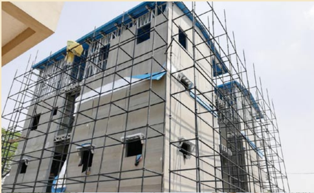
Bihar Shariff, Bihar [36 DUs (G + 2)] using Structural Stay in Place Formwork System (Coffor) – Structural work completed, finishing work in progress.
