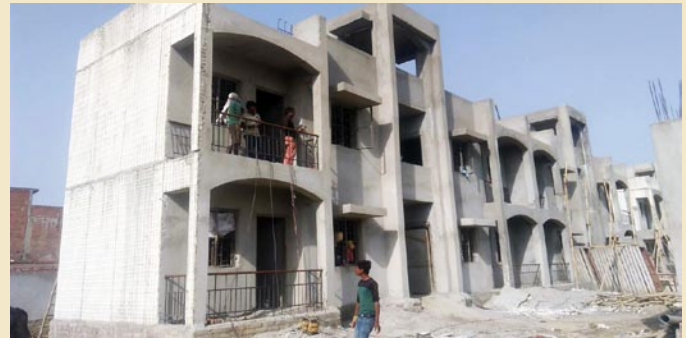
Aurangabad Jagir, Lucknow, Uttar Pradesh [40 DUs (G + 1)] using Stay in Place EPS based double walled panel System (Sismo) – Structural work completed, finishing work in progress.
