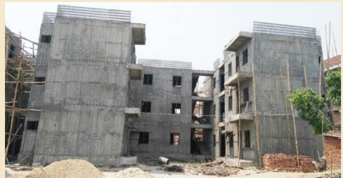
Bihar Shariff, Bihar [36 DUs (G + 2)] using Structural Stay in Place Formwork System (Coffor) – Structural work completed, finishing work in progress.
