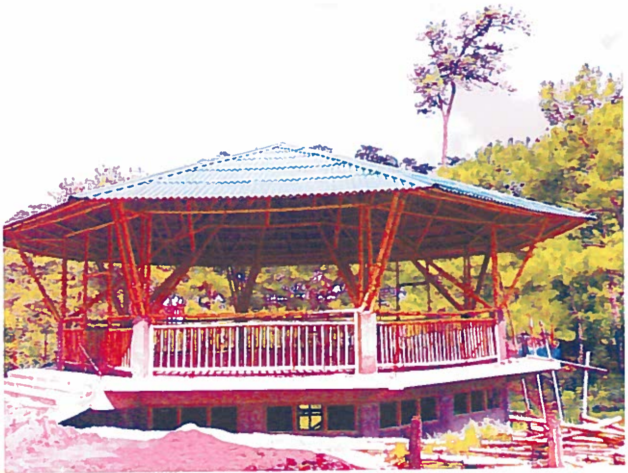
Bamboo Demonstration Structure at Aurvindo ashram, Shillong
