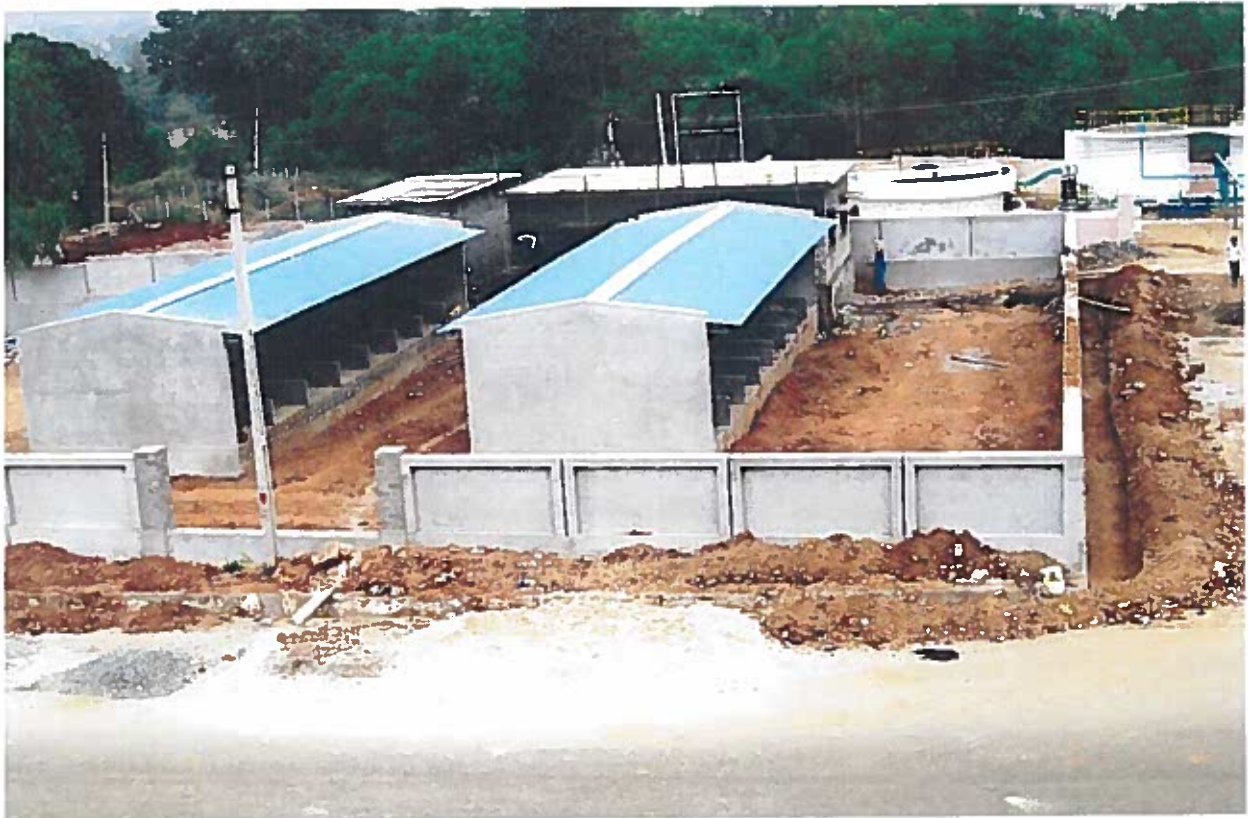
Demonstration Informal Market being constructed by BMTPC at Vishakhapatnam, Andhra Pradesh
