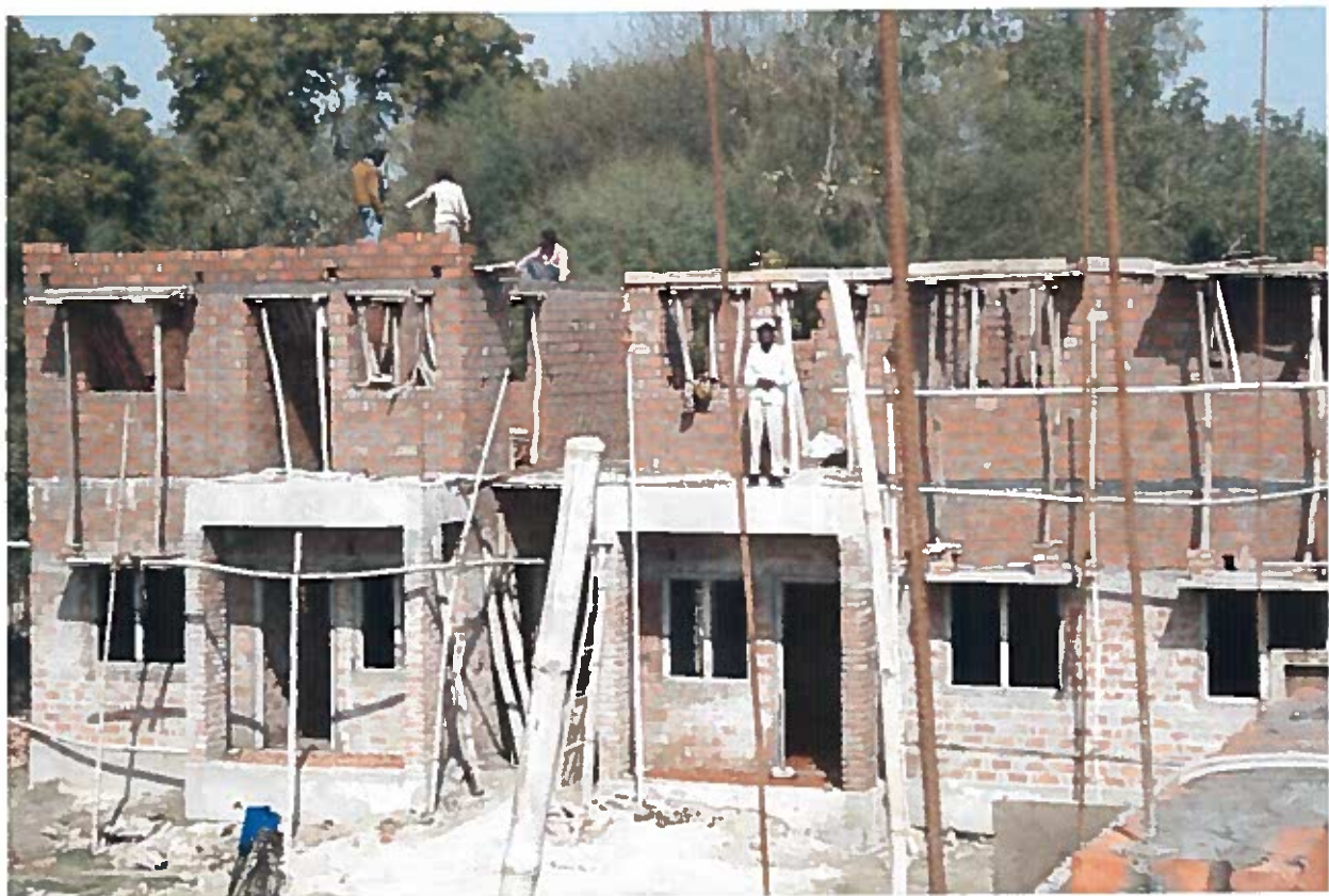
Demonstration Houses being constructed by BMTPC at Amethi, Sultanpur, Uttar Pradesh
