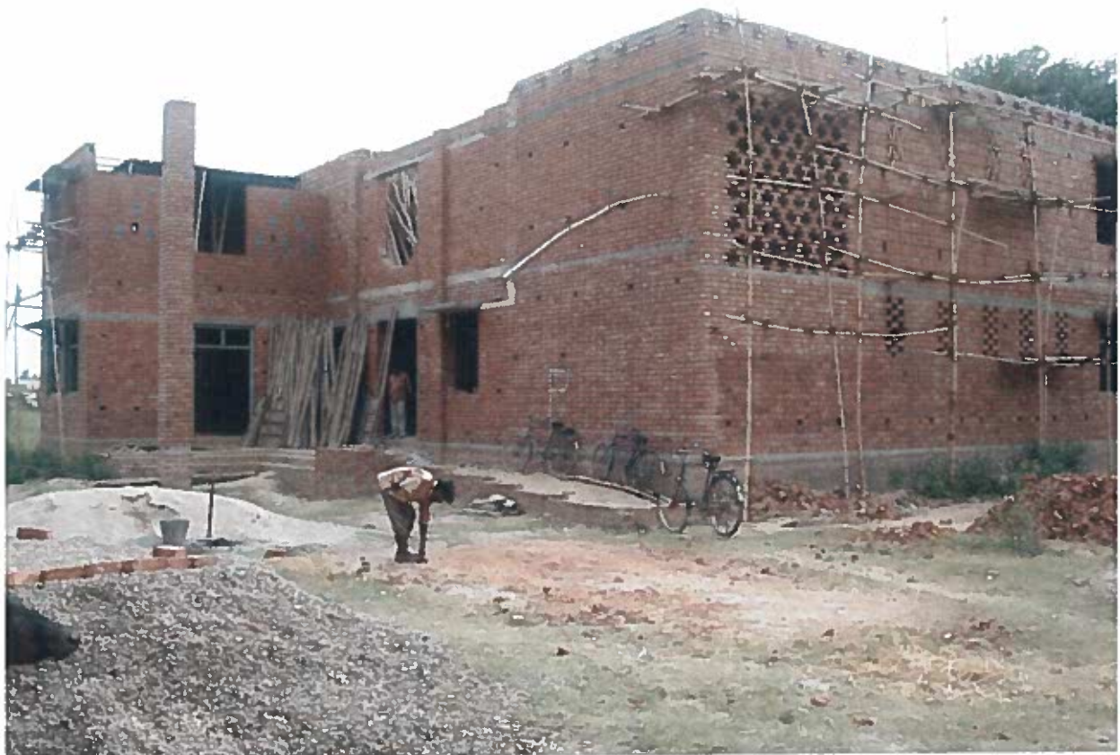
Demonstration Community Centre being constructed by BMTPC at Village Khojkipur-Naggal, Haryana
