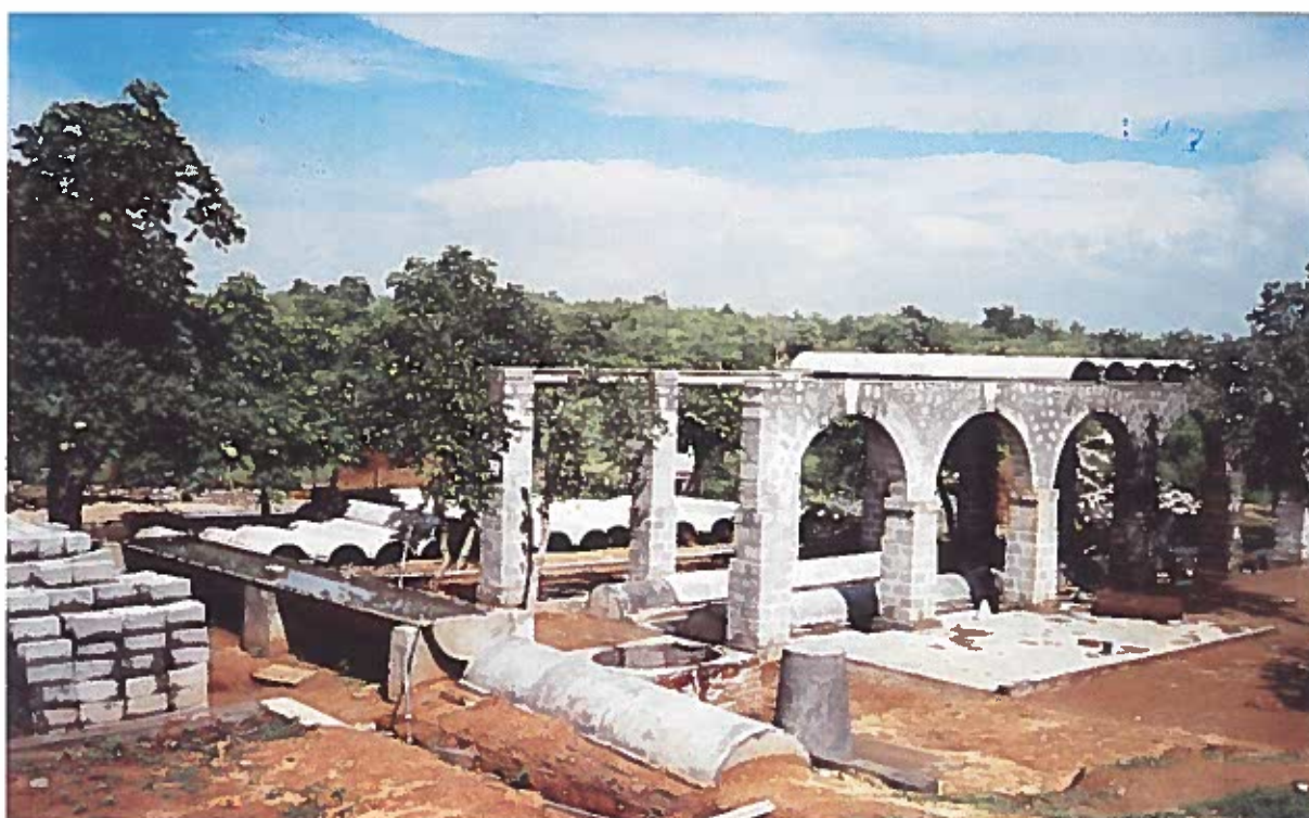
A shed constructed with Ferrocement Roofing Channels
