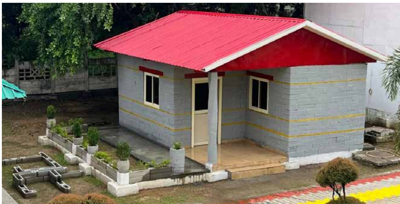
3D Printed House using Agro-waste based Modular Hollow Blocks at CBRI Roorkee
