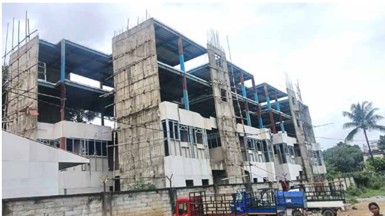
Demonstration Housing Project (for Contractual Safai Karamcharis) and Community Centre under PMAY(U) using Light Gauge Steel Structural System – LGSF with V-infill Wall at Guwahati, Assam
