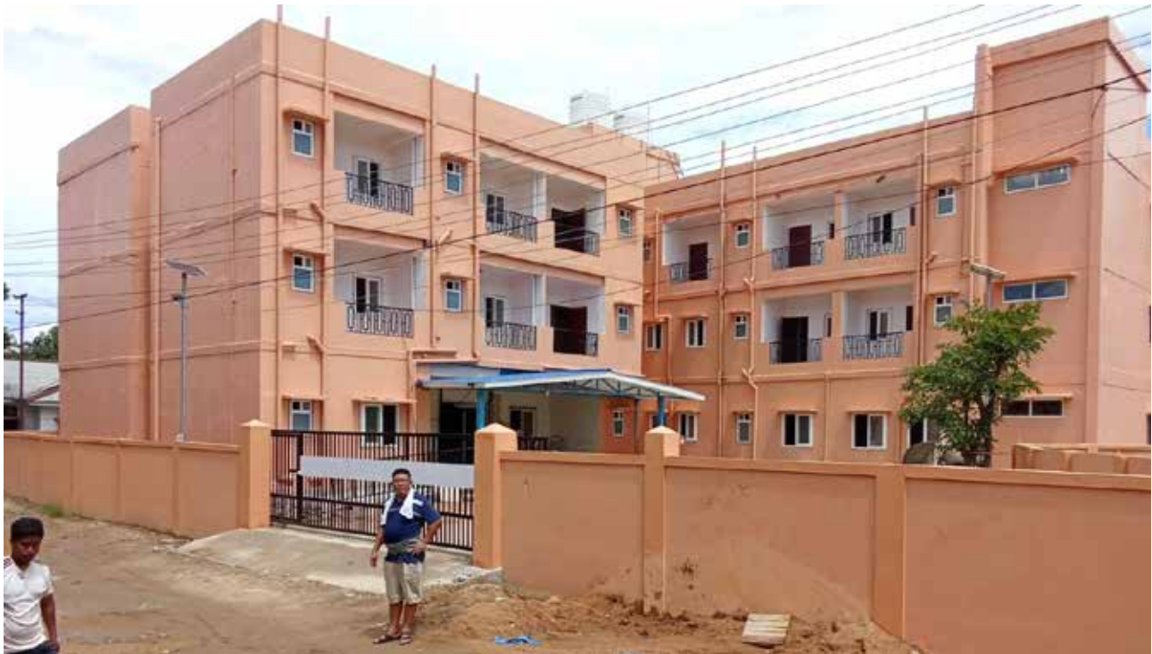
Demonstration Housing Project (Working Women Hostel) and Community Centre under PMAY(U) using Prefabricated Sandwich Panel system – EPS Cement Sandwich Panels with Steel Structure at Dimapur, Nagaland
