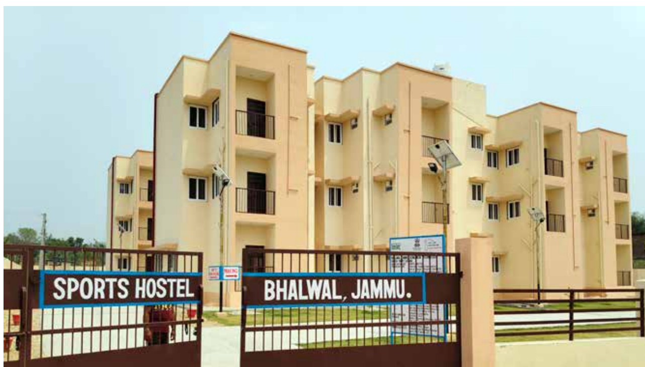
Demonstration Housing Project (Sports Hostel) under PMAY(U) using Prefabricated Sandwich Panel System – EPS Core Quik Build Panels at Bhalwal, Jammu, J&K
