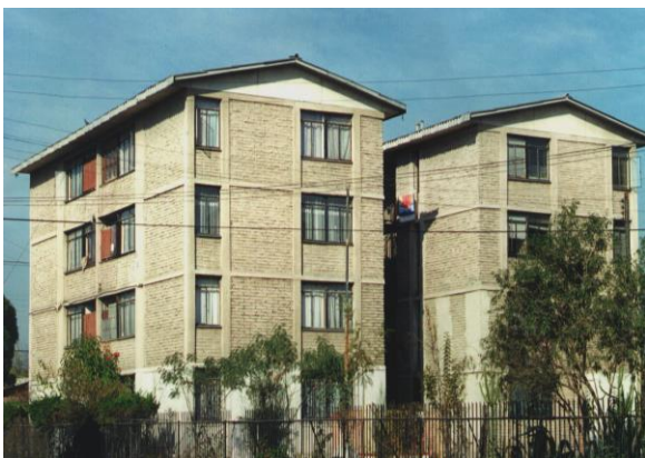
Figure 1: Confined Masonry Construction – (a) components of CM system, and (b) 4-storey house constructed in Chile with CM system.
