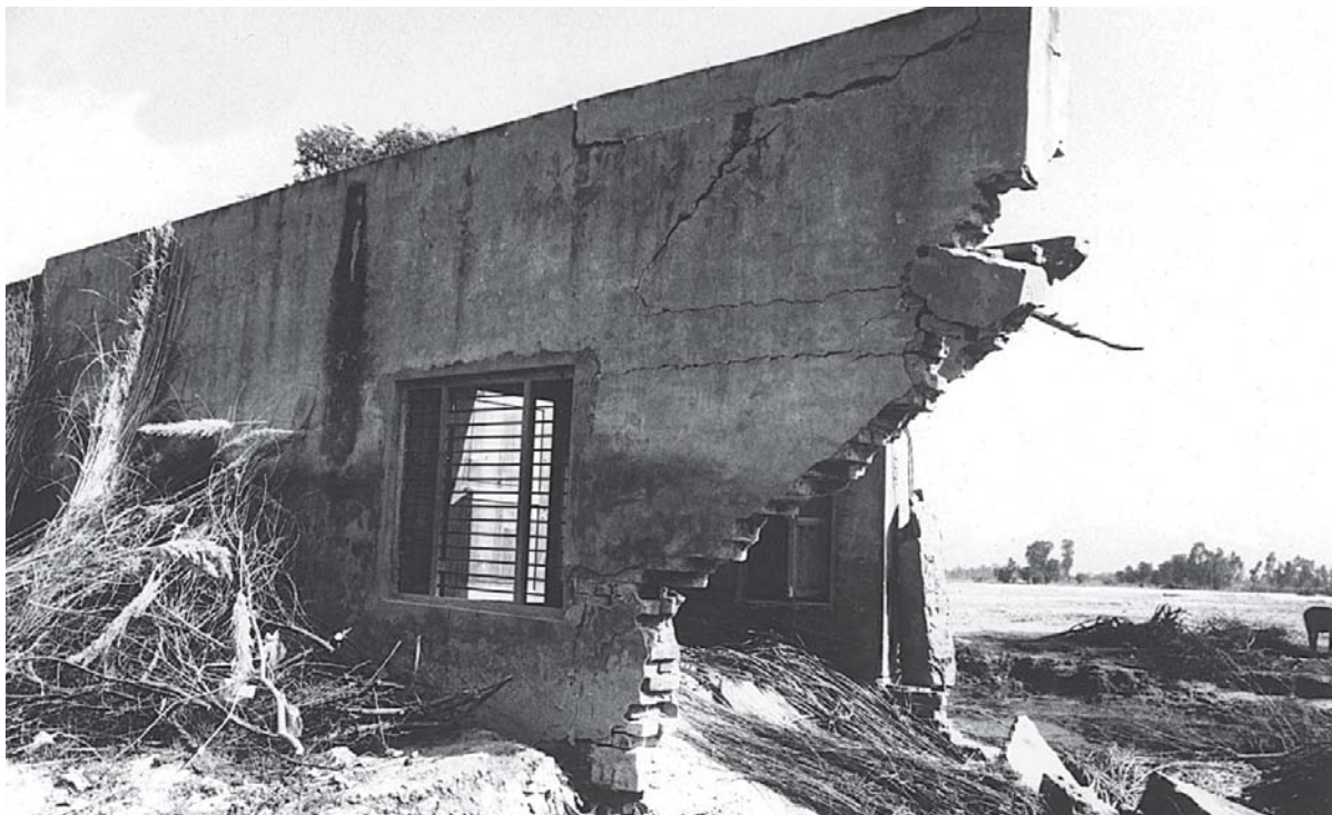
Fig. 4: High velocity of flood water leading to wall collapse due to under scouring
