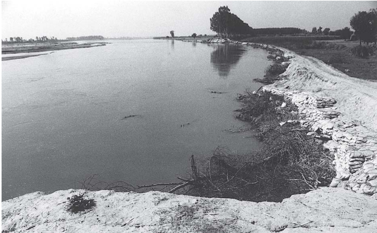
Fig. 2: Breaching at the Embankment of Sutluj
