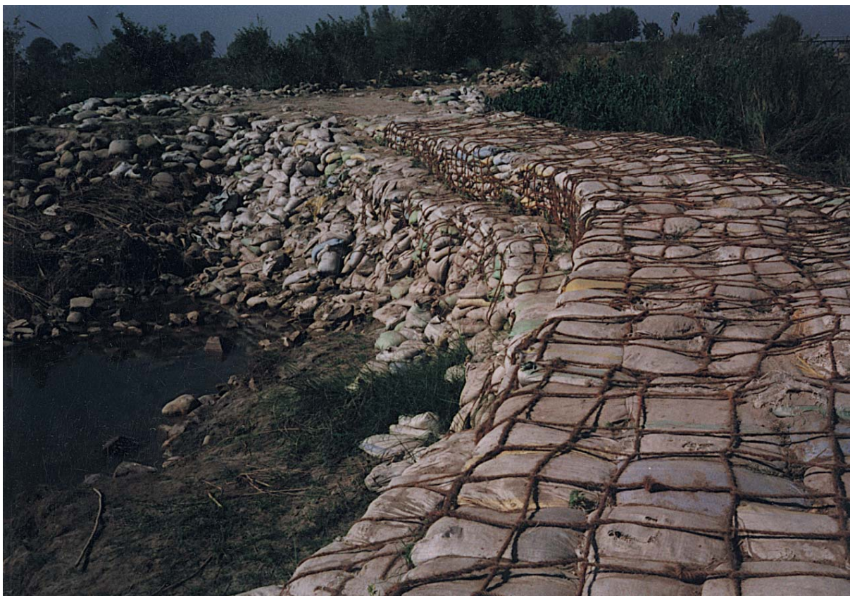
Fig. 3: Plugging of Breach with Sand Bags
