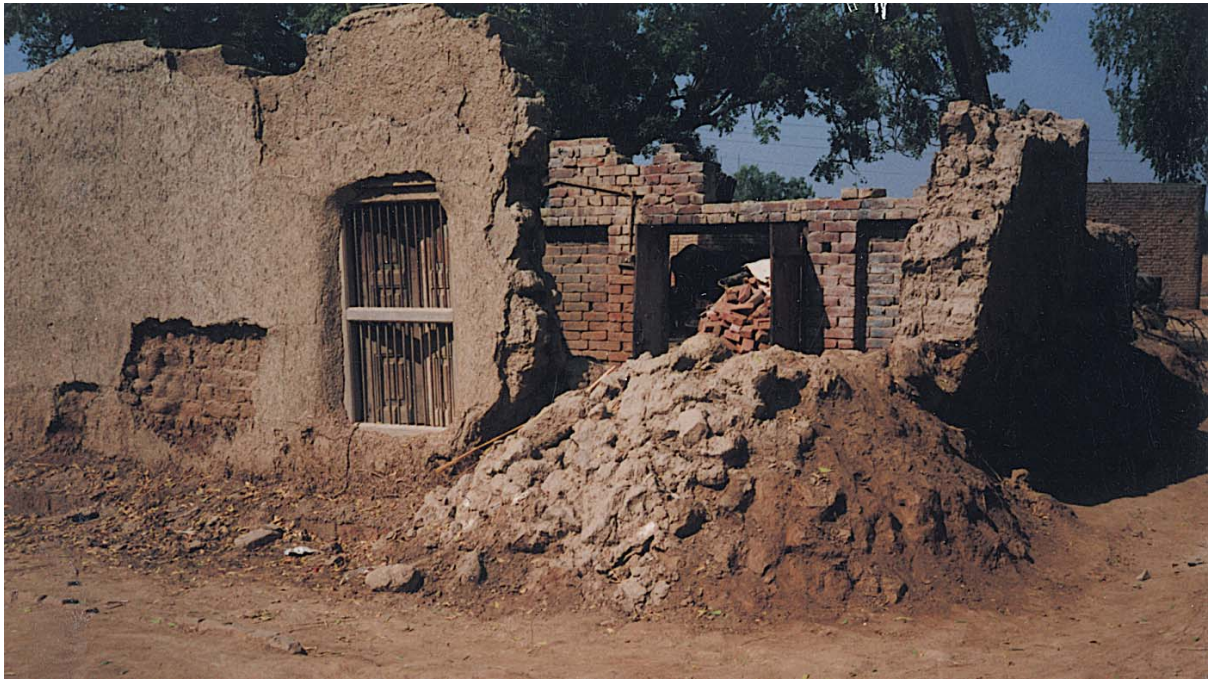
Fig.5: Collapse of earth roof building due to saturation
