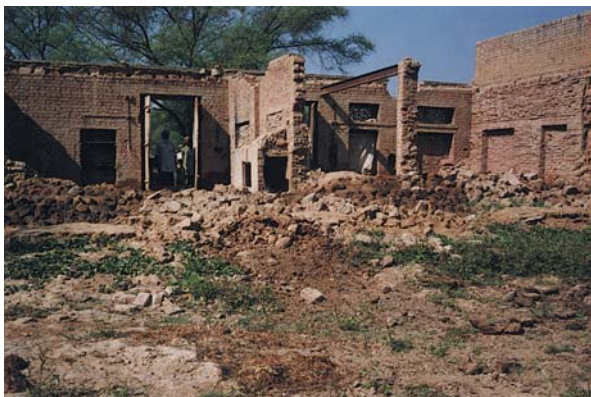
Fig.6: Collapse of tile roof building due to inundation
