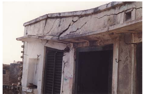
Fig. 7: Extensive cracking of the walls due to differential settlement
