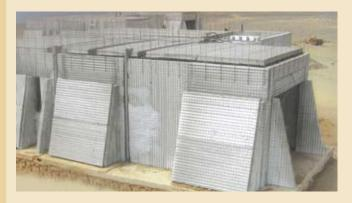
Once the panels are installed as per the requirement of the building, they are anchored and finished with the application of light concrete on both of their sides.
