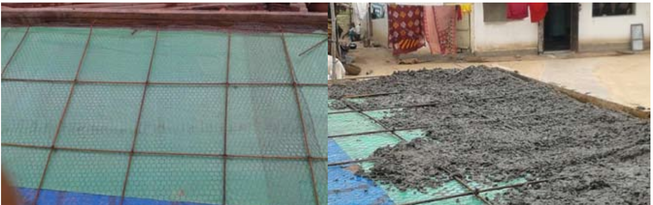
Figure 8(a,b) Rod binding and casting the roof
