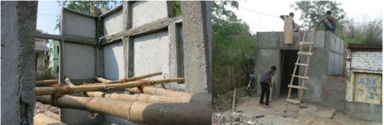
Figure 7(a,b) The continuous top layer and roof shuttering
