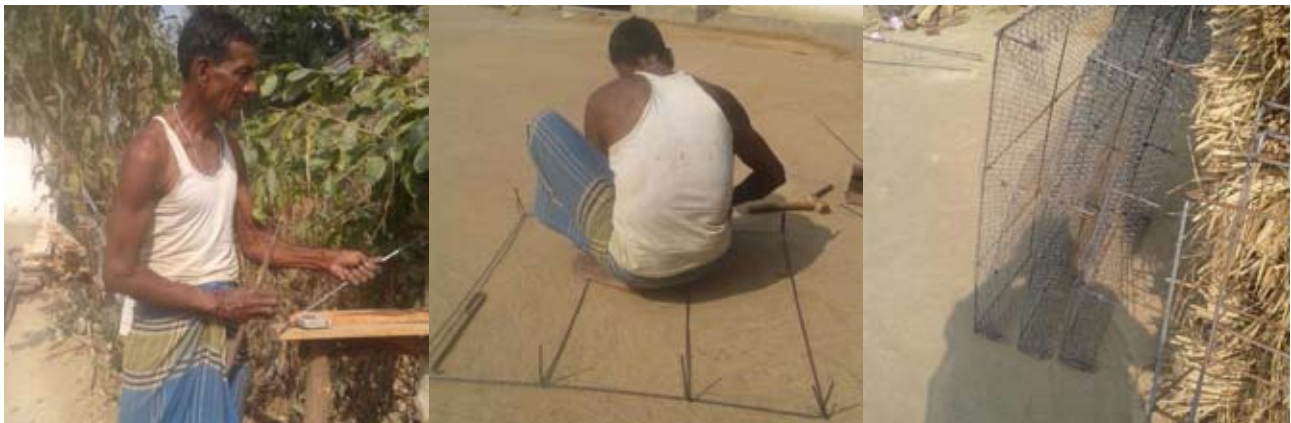
Figure 2(a,b,c) Making of the framework by the mason
