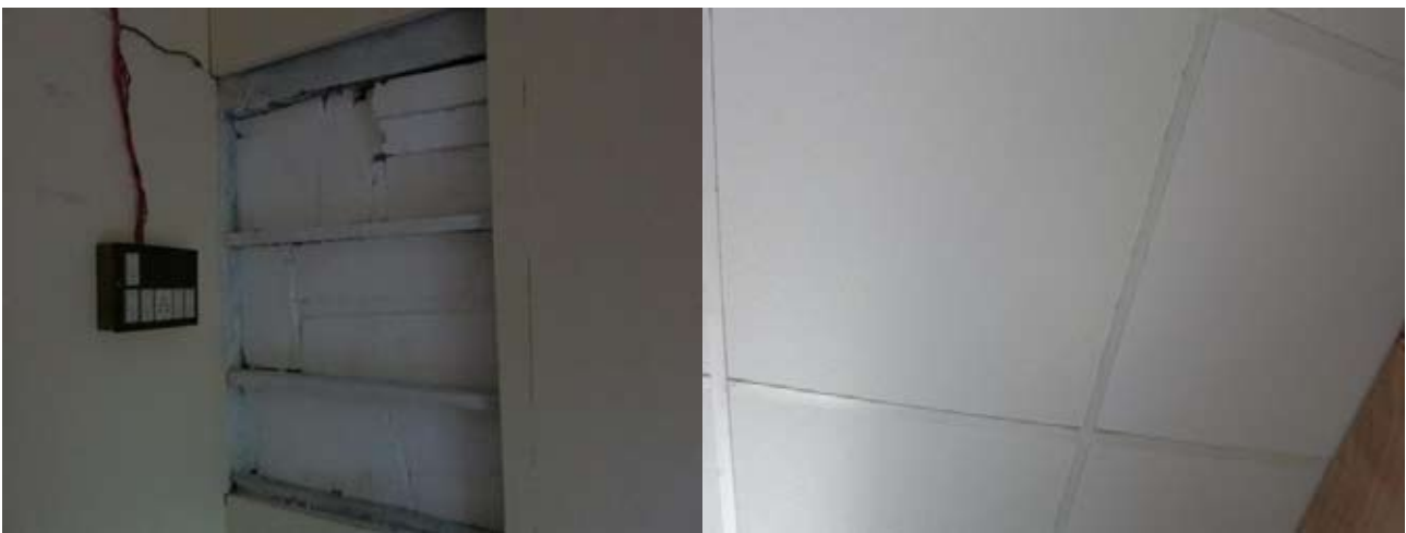
Figure 12(a,b) Plywood covering over thermocol set within the panels and false ceiling on roof
