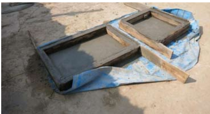
Figure 3. Casting of the wall panel
