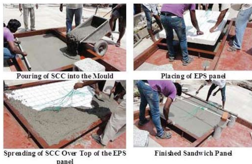
Fig.2 Casting Sequence of Sandwich Panel
