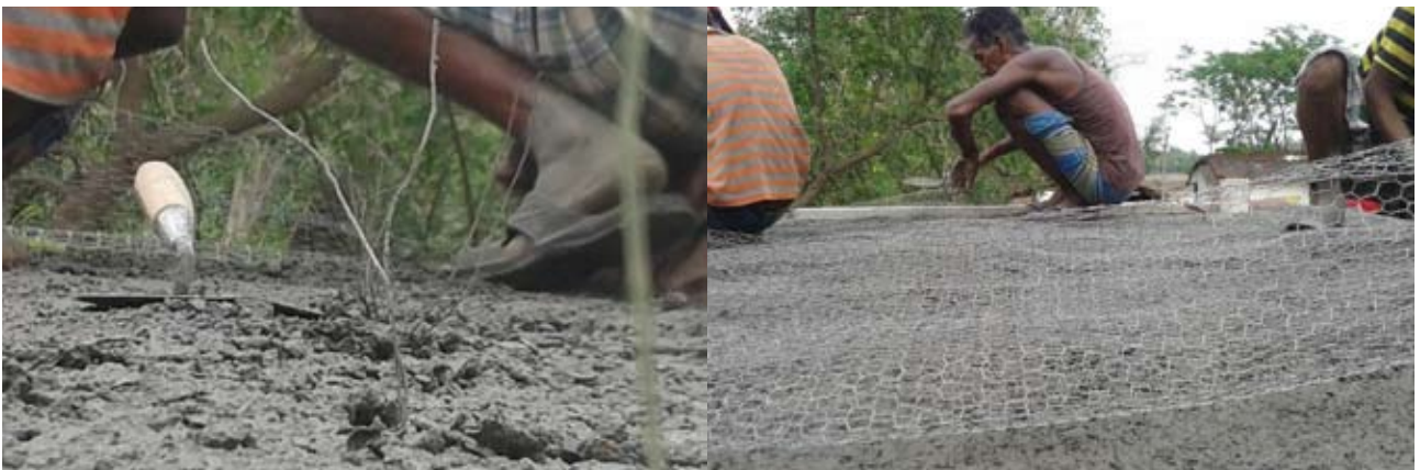
Figure 9(a,b) Laying the second layer of wire mesh
