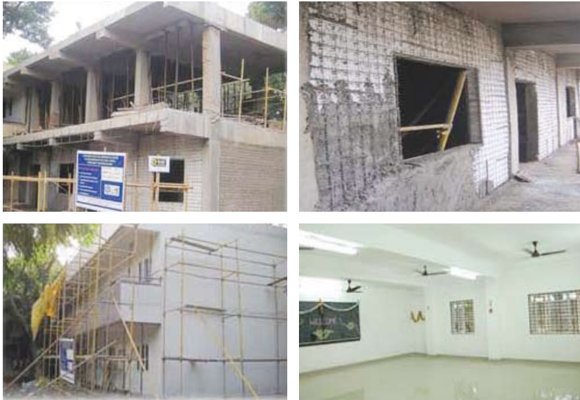
Fig.10 KV CLRI School Building with Light Weight Panels using EPS
