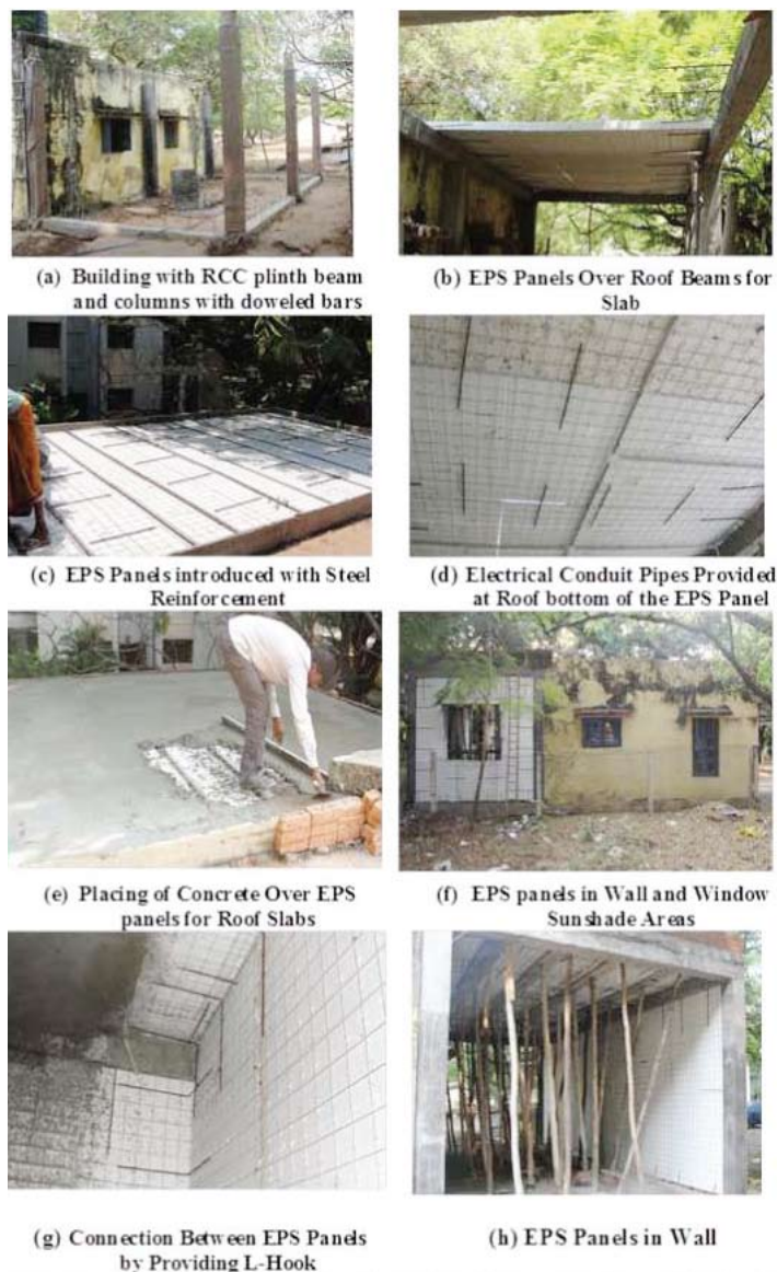
Fig.8 Crèche Building at CLRI with Light Weight Panels both on Walls and Roofs
