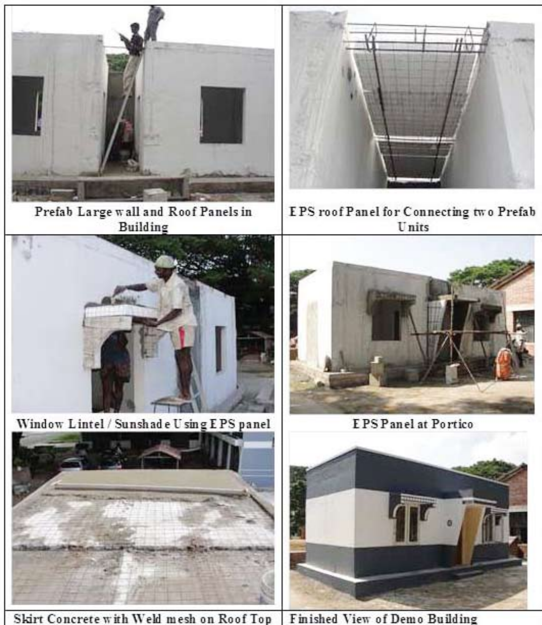
Fig.9 Construction Sequence of Demo Building with Prefab Wall and Roof Panels using EPS
