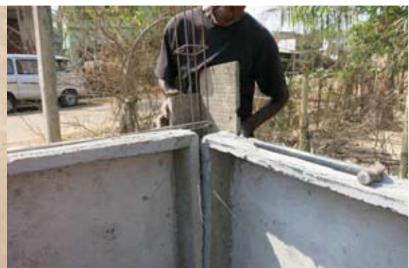
Figure 4. Placing the panel at corner
