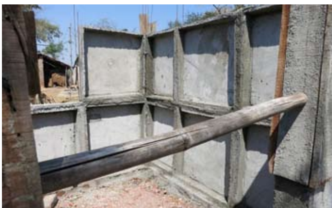
Figure 6(a,b) Door and window opening and its spanning by integrated lintel with horizontal band
