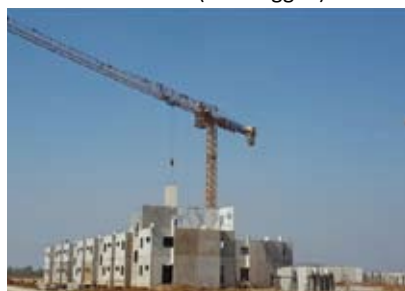
PMAY(U) Houses built with Precast Concrete Technology in Chhattisgarh
