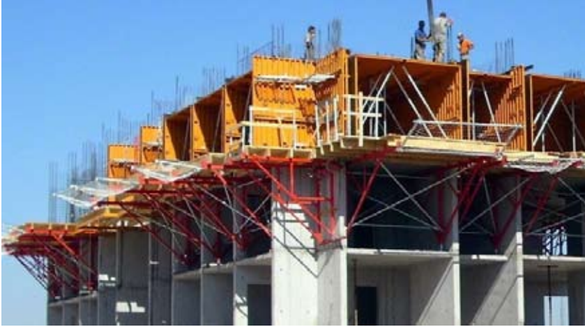
Modular tunnel form work
