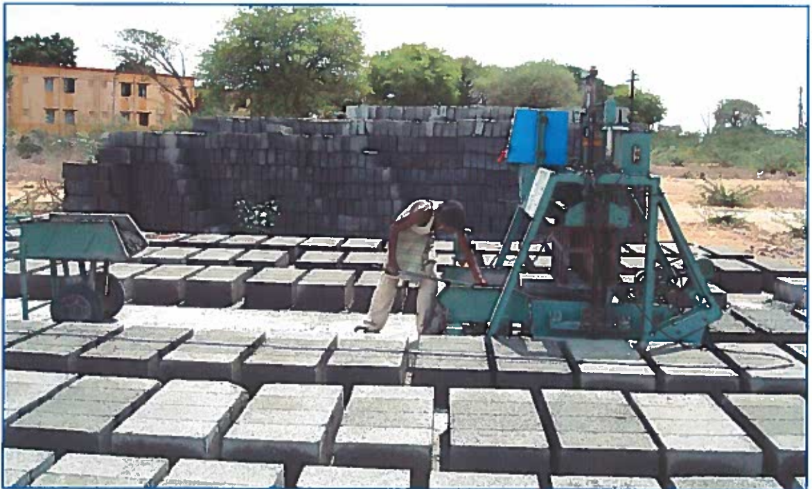
On-site production of Flyash Blocks during the construction of Demonstration Houses under VAMBAY at Trichi, Tamil Nadu
