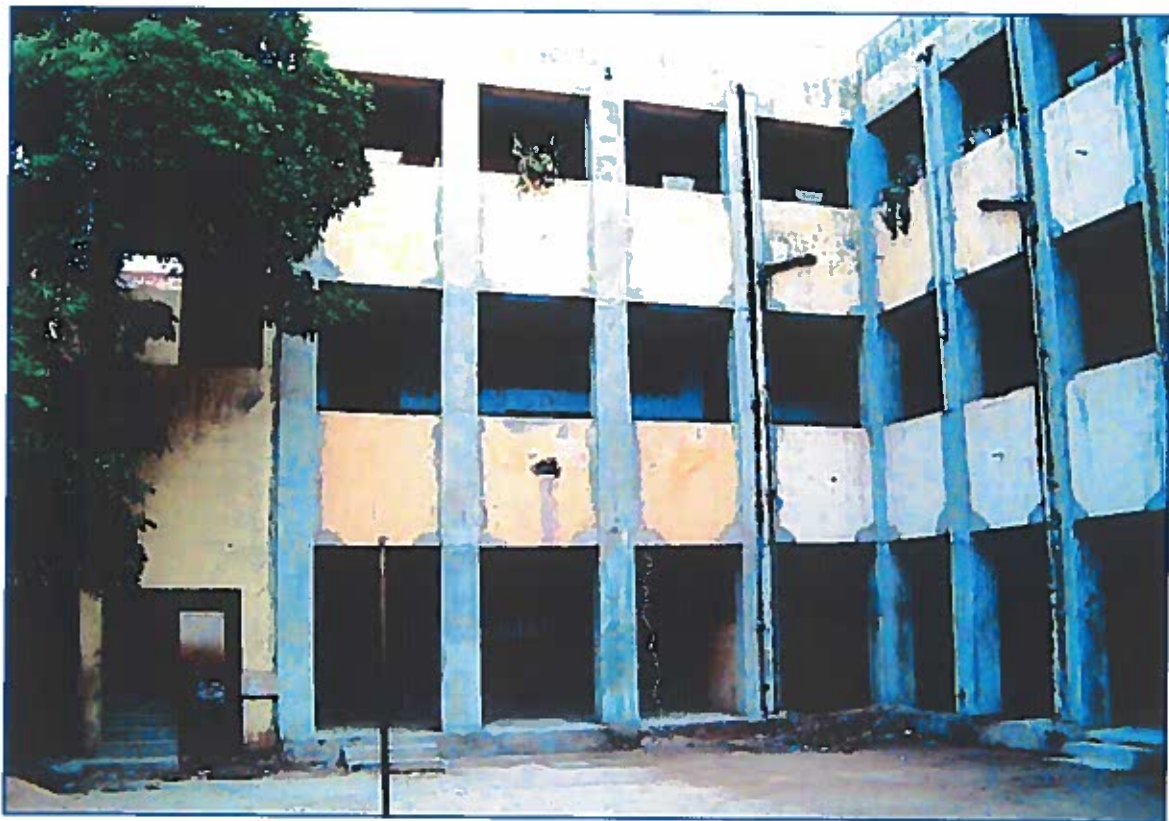
MCD School Buildings retrofitted by BMTPC for seismic strengthening.
