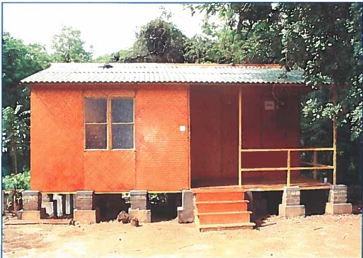
BMTPC designed and developed a pre-fabricated modular housing system using bamboo and bamboo based composites at IPIRTI Bangalore.
