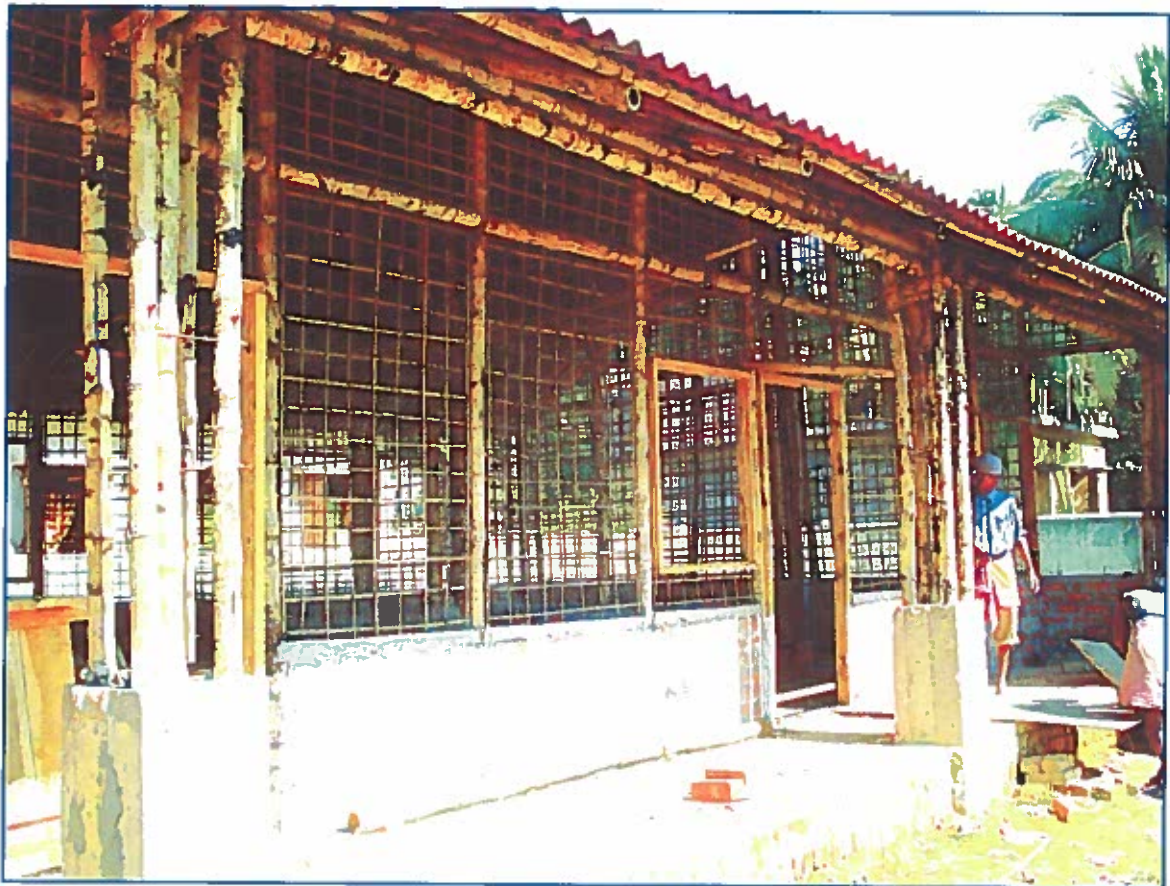
Demonstration School Building at Agartala, Tripura being constructed by BMTPC using bamboo based technologies.
