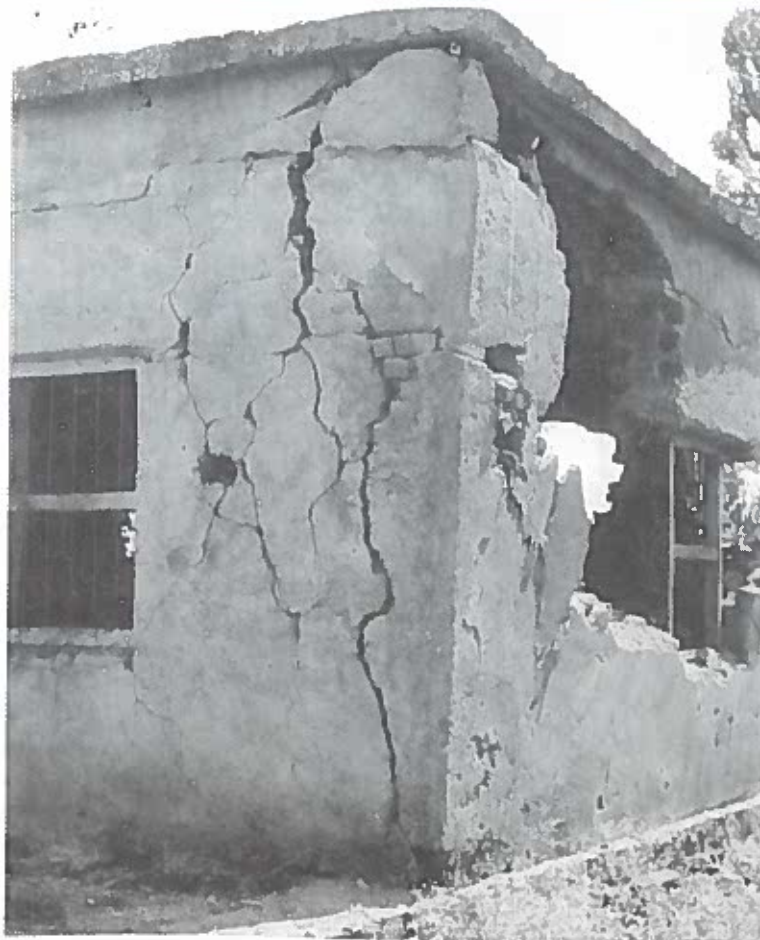
Typical damages during the earthquake in the regions of Maharashtra and Karnataka on 30th September, 1993.
