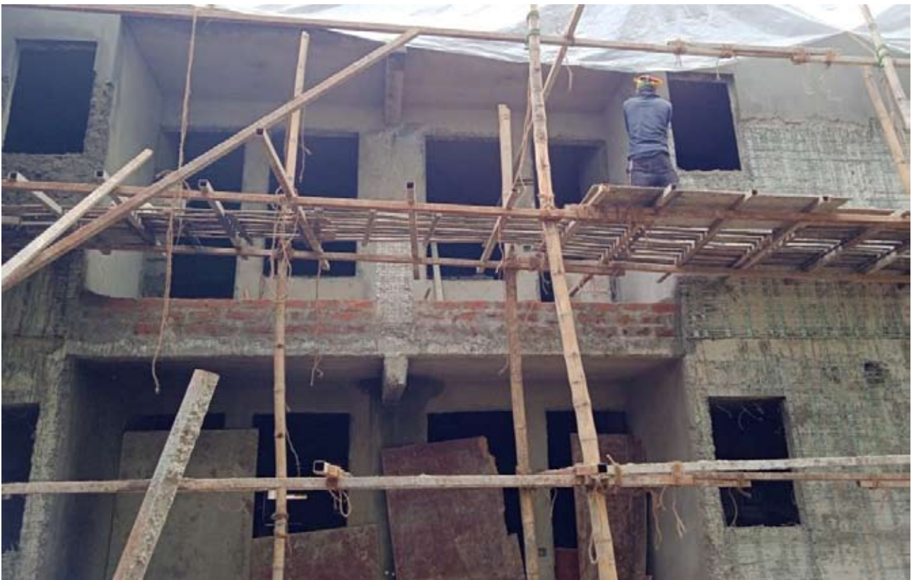
Demonstration Housing Project at Agartala, Tripura using Structural Stay In Place Steel Formwork (Coffor)
