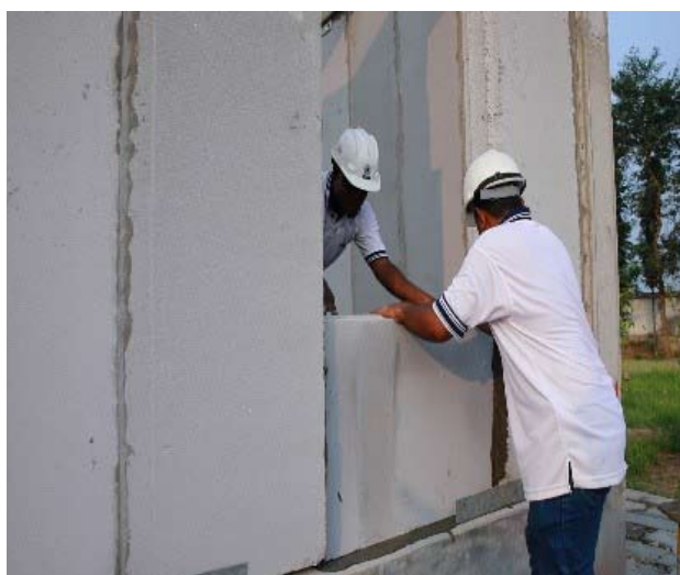
KON_CRETE Reinforced Autoclaved Aerated Concrete (AAC) Panels
