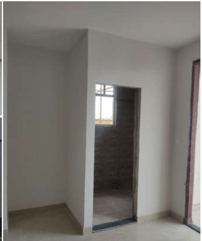
Demonstration Housing Project at Panchkula, Haryana using Light Gauge Steel Framework System (LGSFS) with Cement Fibre board on both side of walls and infill of rock wool
