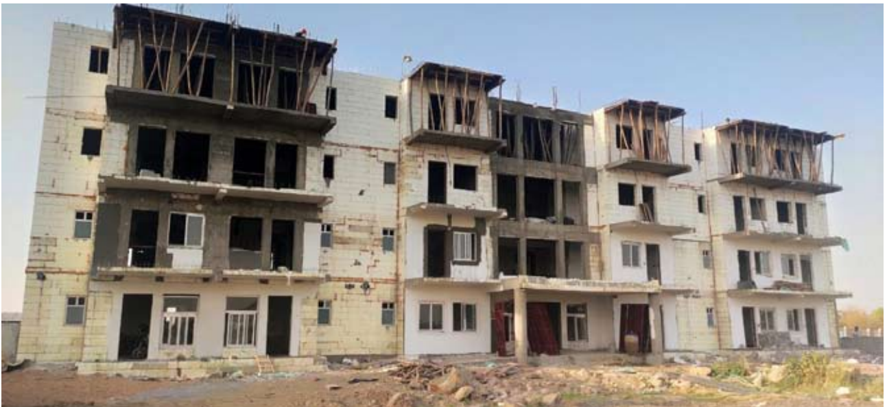
Construction work in progress in Demonstration Housing Project at Bhopal, Madhya Pradesh using Load bearing Monolithic Walls using Insulating Concrete Forms (ICF) Block
