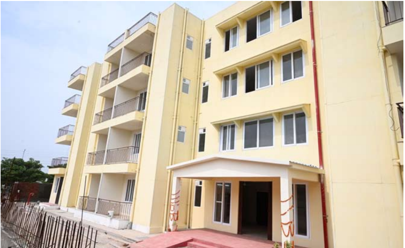
Demonstration Housing Project (Working Women Hostel) under PMAY(U) constructed by BMTPC using Light Gauge Steel Framework System (LGSF) with Fibre Cement Board on both side and infill of rock wool at Panchkula, Haryana
