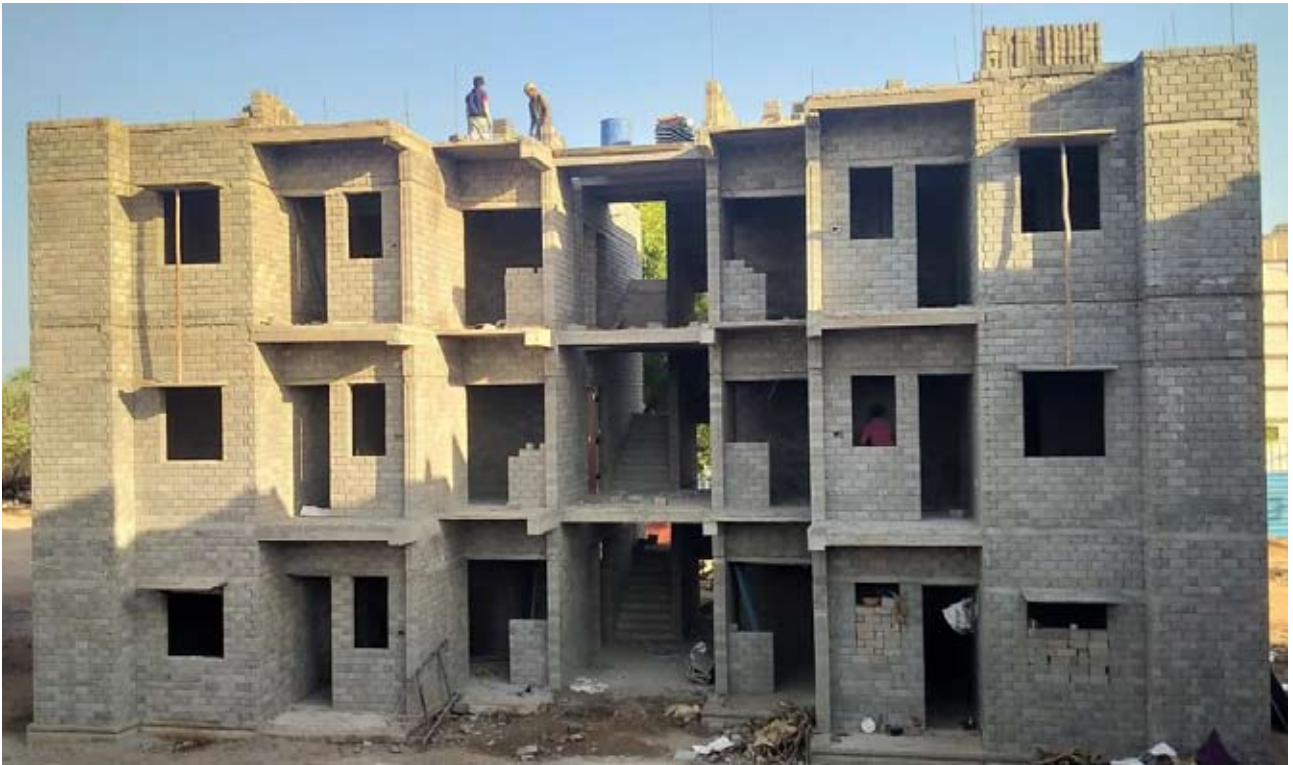
Construction work in progress in Demonstration Housing Project at Ahmedabad, Gujarat using emerging technology - Integrated Hybrid Solution-One
