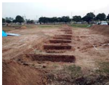
Excavation of foundation at pits at Demonstration Housing Project being constructed at Panchkula, Haryana using Light Gauge Steel Framework System (LGSFS) with Cement Fibre board on both side of walls and infill of rock wool
