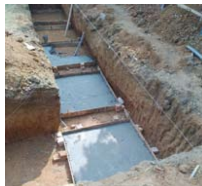
Excavation of foundation pits and laying of PCC at Demonstration Housing Project being constructed at Agartala, Tripura using Structural Stay In Place Steel Formwork (Coffor)
