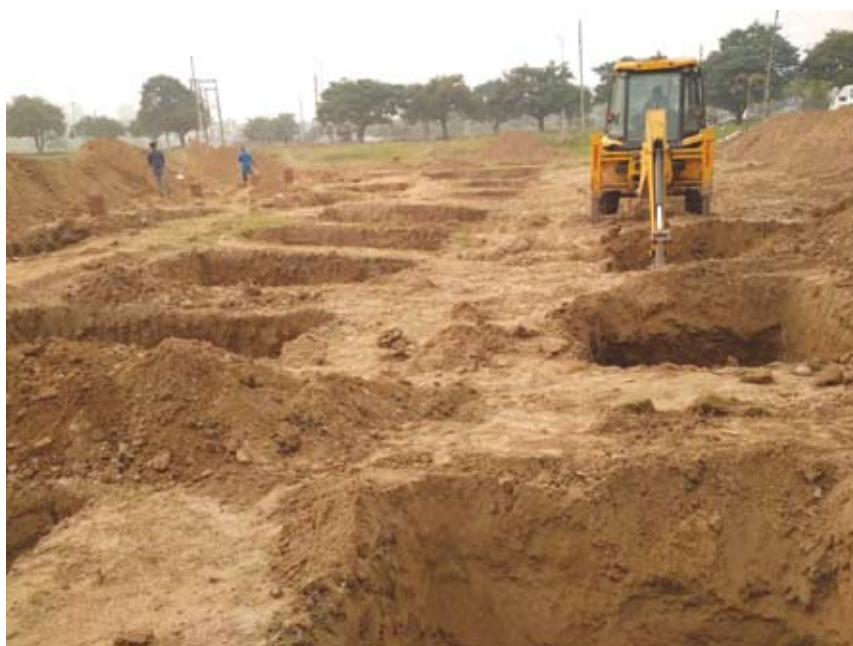
Excavation of foundation at pits at Demonstration Housing Project being constructed at Panchkula, Haryana using Light Gauge Steel Framework System (LGSFS) with Cement Fibre board on both side of walls and infill of rock wool
