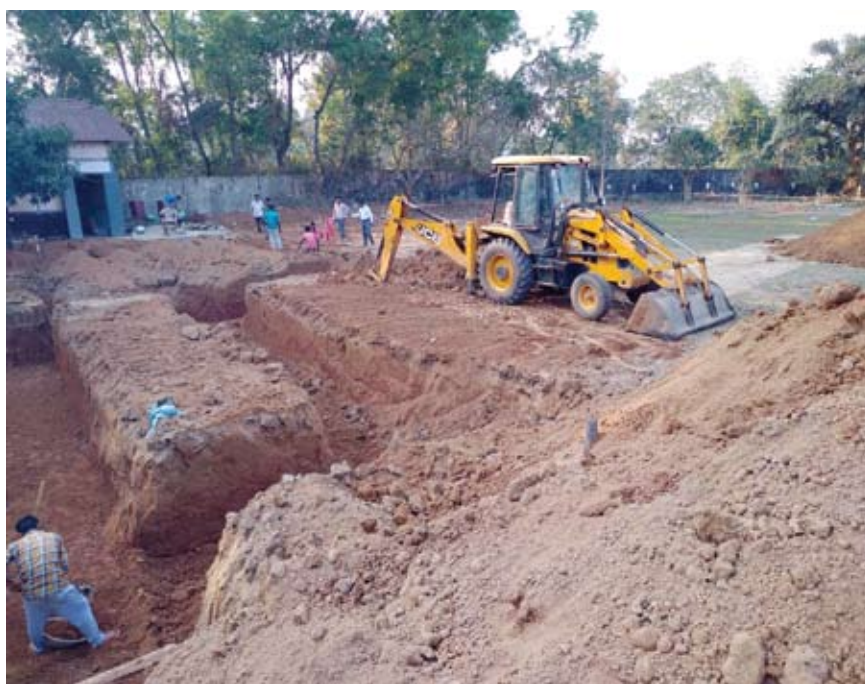
Excavation of foundation pits and laying of PCC at Demonstration Housing Project being constructed at Agartala, Tripura using Structural Stay In Place Steel Formwork (Coffor)
