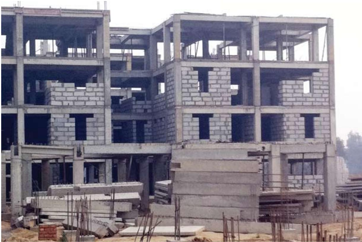
**Emerging Technology - Industrialized 3-S System using Cellular Light Weight Concrete Slabs & Precast Columns**
