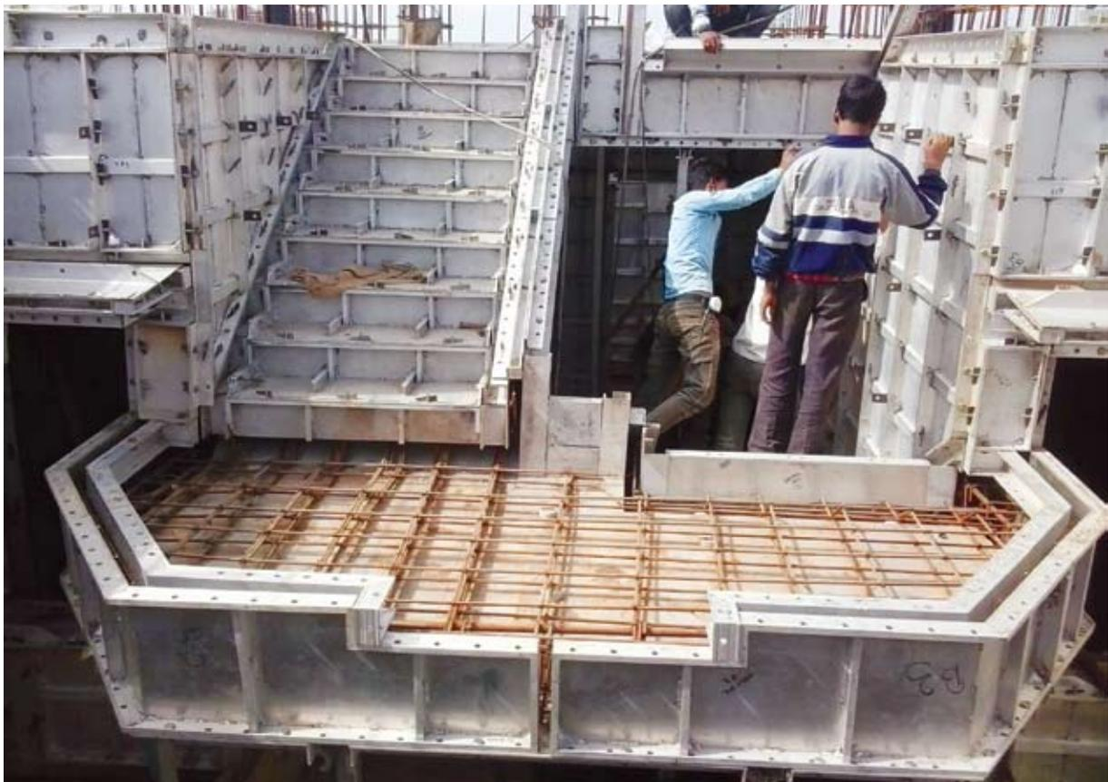
**Emerging Technology - Monolithic Concrete Construction System using Aluminium Formwork**
