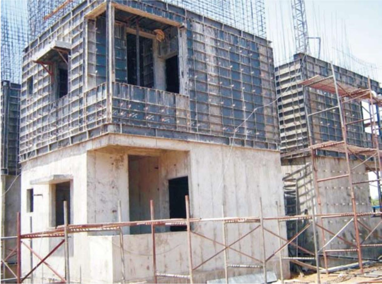
**Emerging Technology - Monolithic Concrete Construction System using Plastic - Aluminium Composite Formwork**
