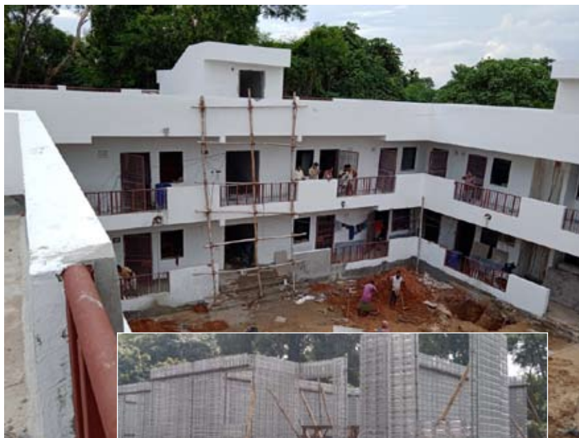
Use of Structural Stay-in-Place Steel Formwork (Coffor) System at Agartala, Tripura
