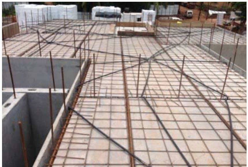
Figure 4 Routing of Conduits in Plan within Screed
