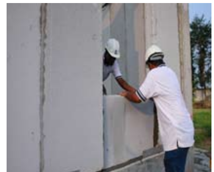
KON_CRETE Reinforced Autoclaved Aerated Concrete (AAC) Panels
