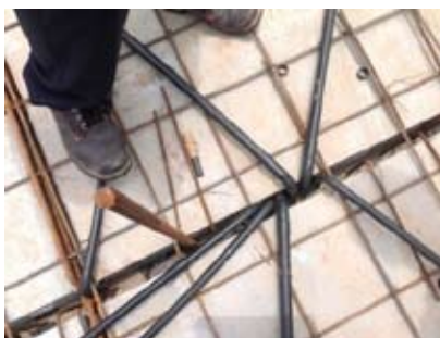
Figure 2 Conduits congestion at DB Box Junction
