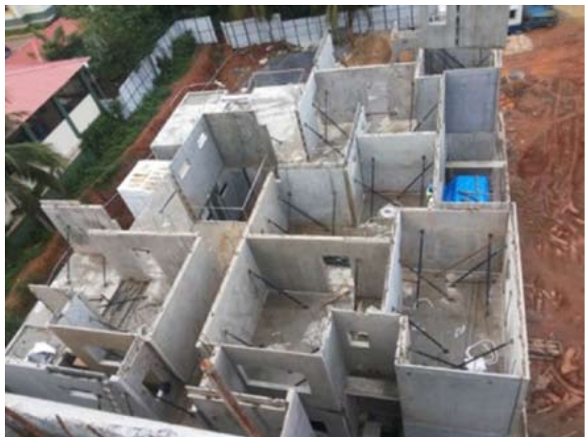
Figure 5 Typical Flat Unit : Erection In Progress
