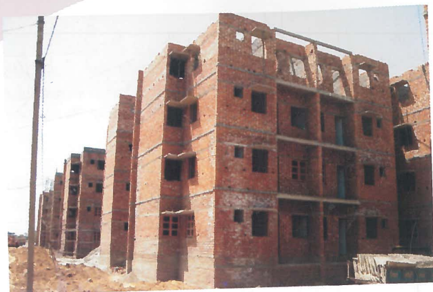
Brick Load Bearing Construction
