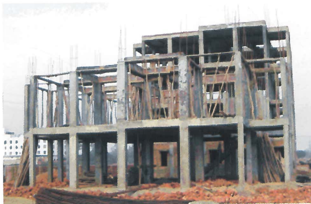
RCC Framed Construction
