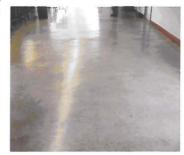
The base concrete, either in cement or lime, about 7.5 to 10 cm
