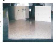
For a 40 mm thick Terrazzo floor an under layer of concrete 34 mm thick is first provided over the base concrete which is finished with a topping of terrazzo, 6 mm thick. Paneling etc can be done as in the case of cement concrete flooring. The surface obtained after
