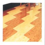
PVC tiles are usually square in shape having sides of 30 cm, 60 cm or 90 cm. Sheets and rolls of PVC are also available for providing larger floors. These tiles are fixed to the floor tops with the help of adhesives, especially recommended for the purpose.
