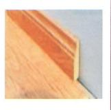
Care should be taken that the skirting is of a uniform thickness and height.
