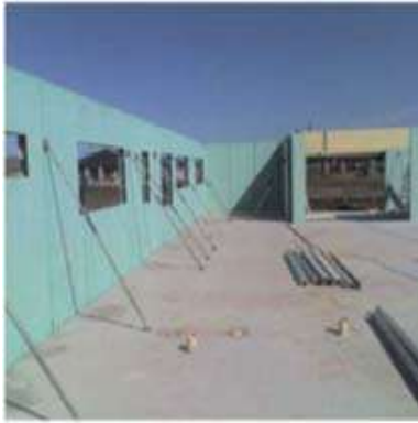
Fig. 8 Diagonal bracing Fig. 9 Corner connection
