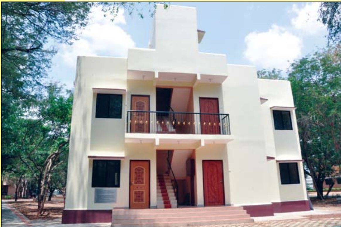
Constructed at IIT Madras Campus in one month duration.
