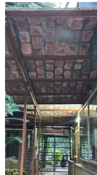
CSEB-Concrete composite: beams, columns and lintels
