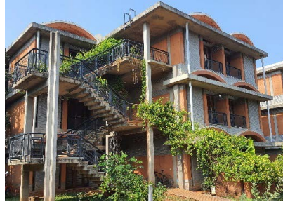
Poured earth concrete
