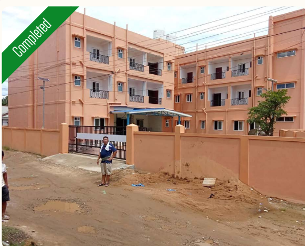
DHP at Dimapur, Nagaland using EPS Cement Sandwich Panels with steel structure
