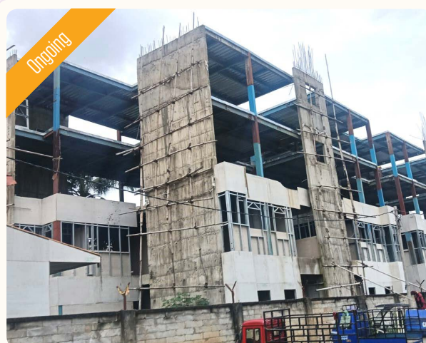
DHP at Guwahati, Assam being constructed using Light Gauge Steel Framework System (LGSFS) with V-infill walls and Pre-engineered Building (PEB) steel structure
