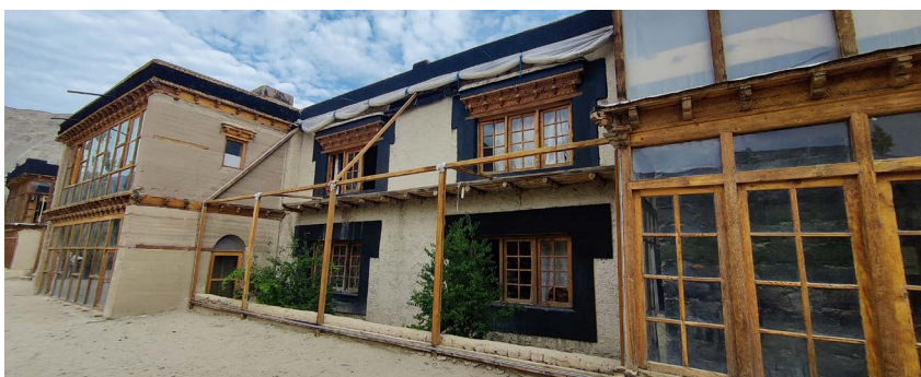
Rammed Earth Construction
