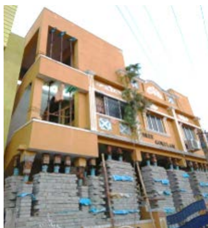
Building Lifting Technique
