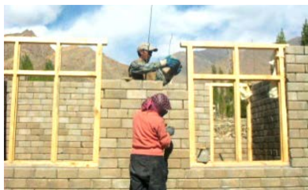
Fig. 4: Houses in Ladakh: Engineered Houses with local soil using stabilizers like cement/lime
