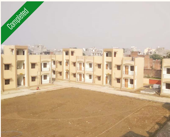
DHP at Lucknow, Uttar Pradesh using Stay in place EPS based double walled panel system with infill concrete
