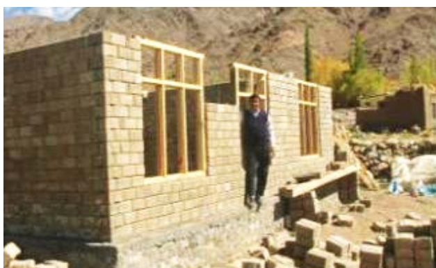
Fig. 4: Houses in Ladakh: Engineered Houses with local soil using stabilizers like cement/lime
