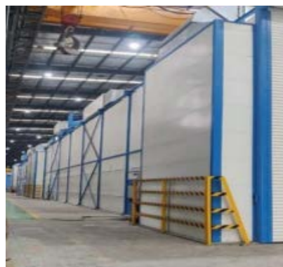
Insulated Sandwich Panel (Rigid Polyurethane/Polyisocyanurate Core)
