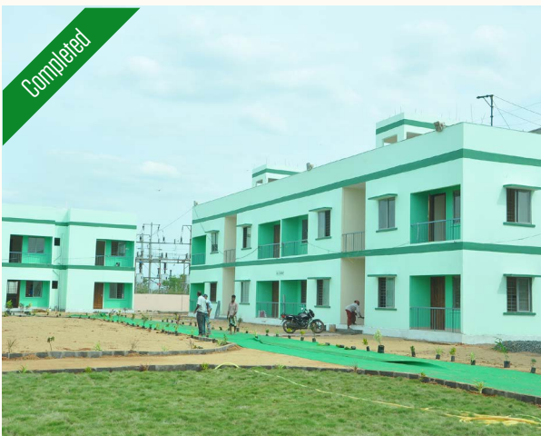
DHP at Nellore, Andhra Pradesh using Glass Fibre Reinforced Gypsum Panel (GFRG) technology for houses and flyash blocks with filler slabs for community building
