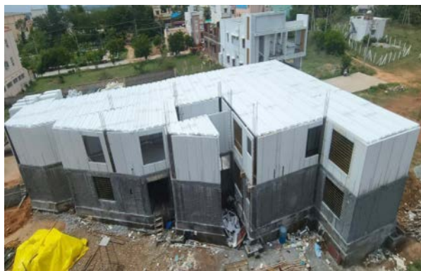
Concrewall - Reinforced EPS Structural Panels (RESP)
