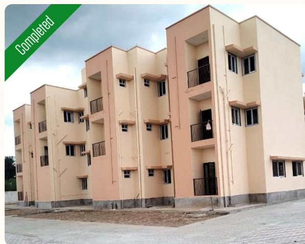
DHP at Bhalwal, Jammu using Prefabricated Sandwich Panel System - EPS core Panel using Quikbuild Panels
