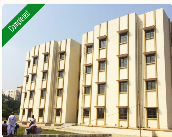
DHP at Bhubaneswar, Odisha using Prefabricated Sandwich Panel System - Reinforced Expanded Polystyrene sheet core with sprayed concrete
