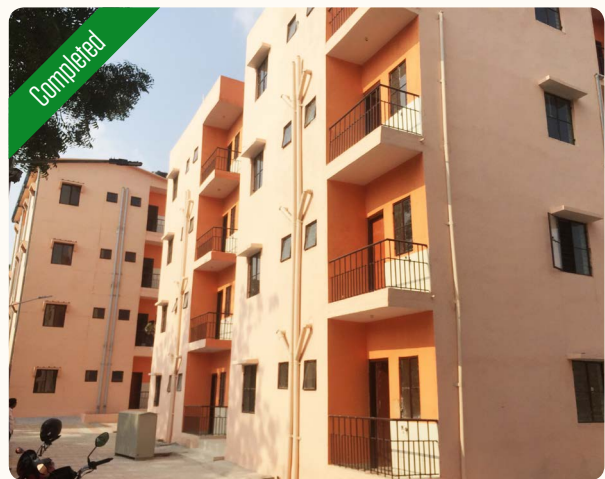
DHP at Hyderabad, Telengana using (i) Structural Stay In Place Steel Formwork System (16 houses) and (ii) Light Gauge Steel Structural System (16 houses)
