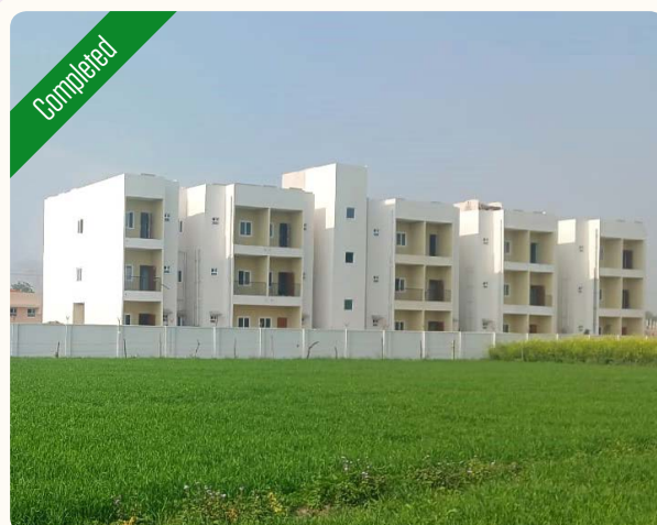
DHP at Ayodhya, Uttar Pradesh using Light Gauge Steel Framework System (LGSF) with Cement Fibre board on both side of walls and infill of rock wool.
