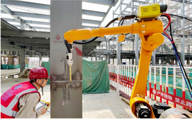
Fig.10: Robotic welding for smarter construction
