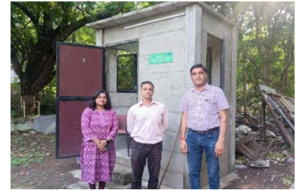
Pre-fabricated Guard Rooms
