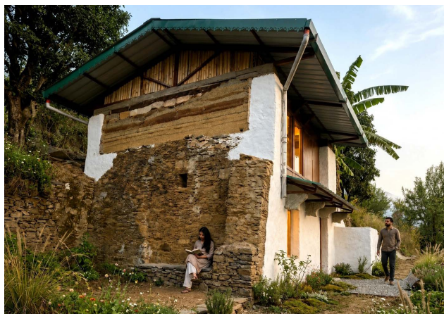
Sunny: a century-old stone room renewed with an interlocking prefabricated hempcrete panel system. Photographs: GoHemp.
