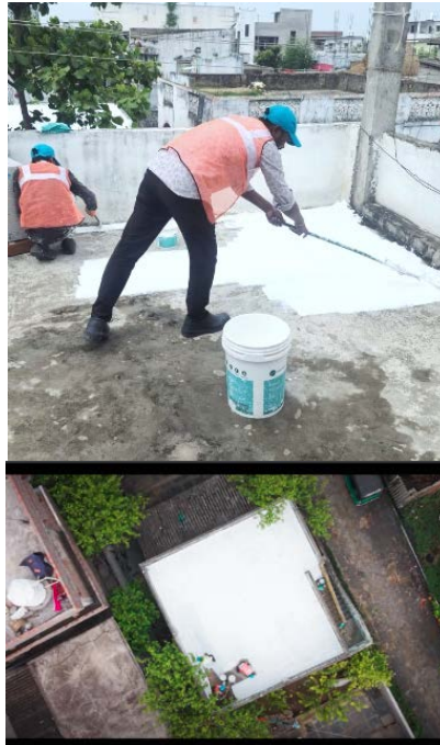
Figure 4: Cool Roof Completed Projects
