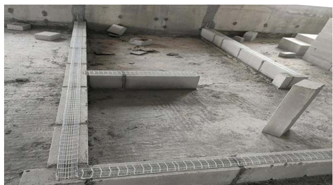
Bed Joint Reinforcement (BJR)
