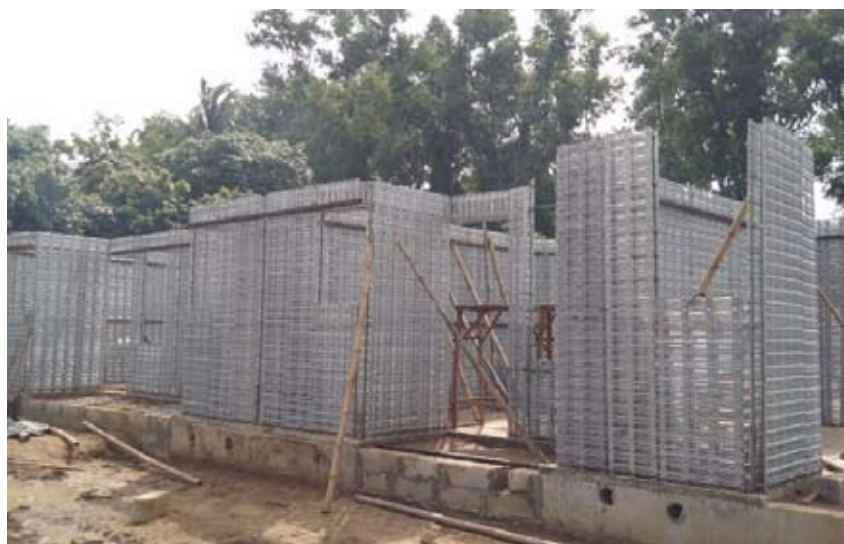
Use of Structural Stay-in-Place Steel Formwork (Coffor) System at Agartala, Tripura
