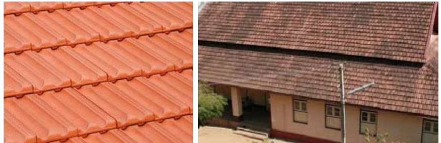
Fig. 6: Mangalore tiles used in roofs (Source -Sarathraj and Somayaji 2014)
