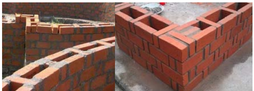
Fig. 9: Rat Trap Bond masonry technique
