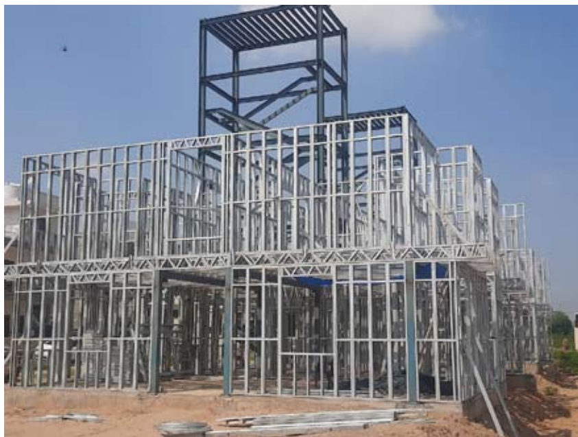
Use of Light Gauge Steel Framework System at Panchkula, Haryana
