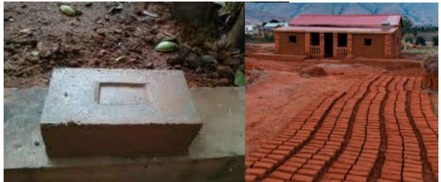
Fig. 8: Adobe Brick wall construction (Source-B. 2014)
