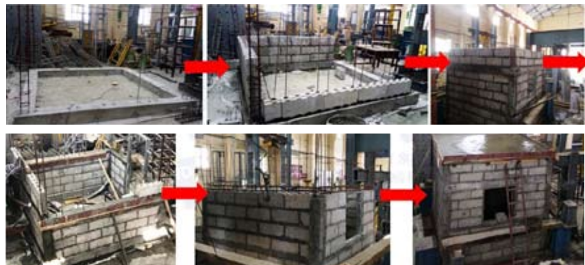
Fig. 3. Construction sequence of CM building using FCC blocks
